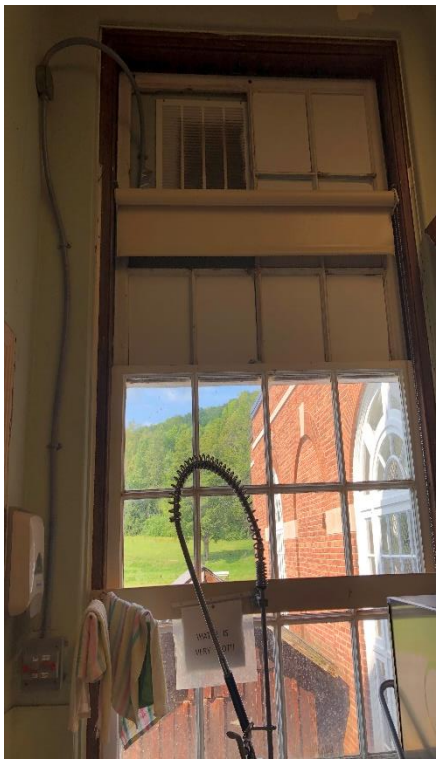
Kitchen exhaust upgrades
