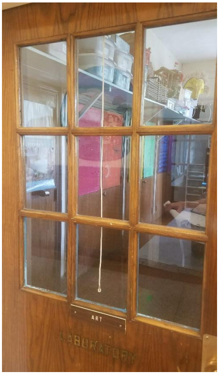
Classroom door replacement
