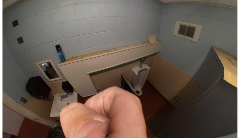
Toilet room ADA upgrades
