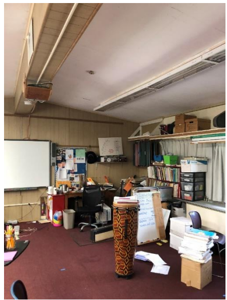
Mech. / Elec. upgrades
