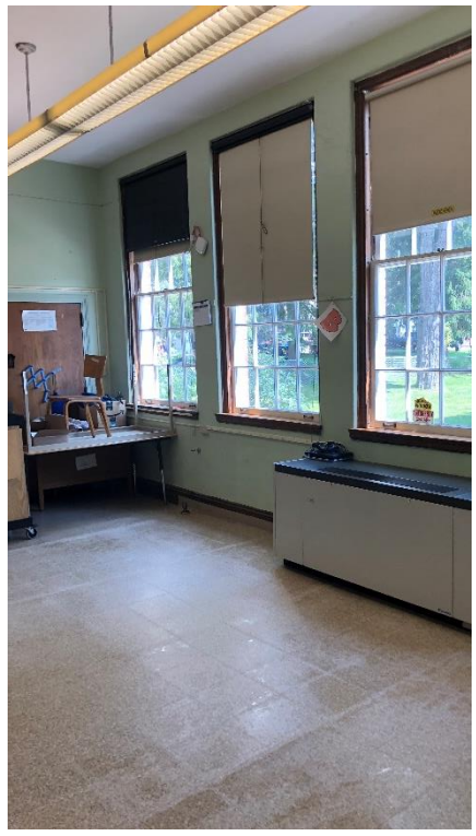
Lighting upgrades & finishes
