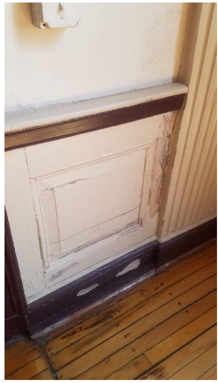
Interior finish repairs
