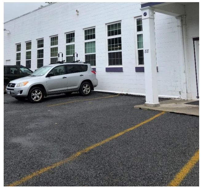
Parking lot improvements
